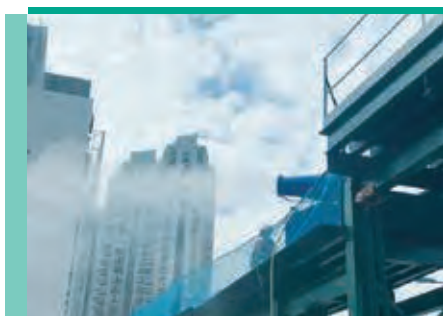
The Group has applied mist cannons for dust suppression. 集團使用霧炮以降低塵埃。
